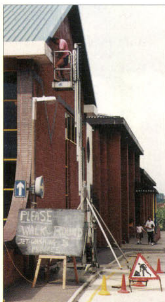
Fig. 1: No...he's not 'jet washing' but using a portable electric drill! This portable American-made telescoping mini-tower could prove useful in antenna maintenance and helps improve safety (see text).
